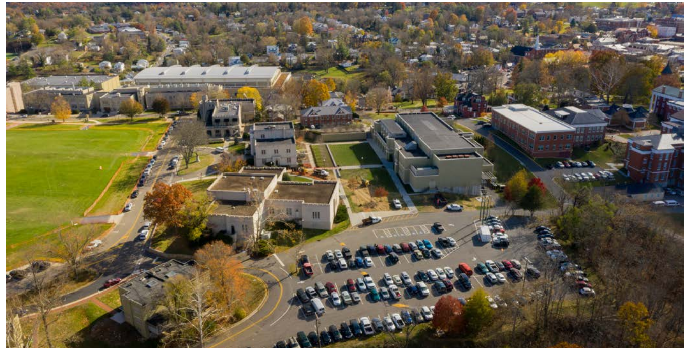
▲ This location for the new facility will create more integration between leadership and daily activities.
