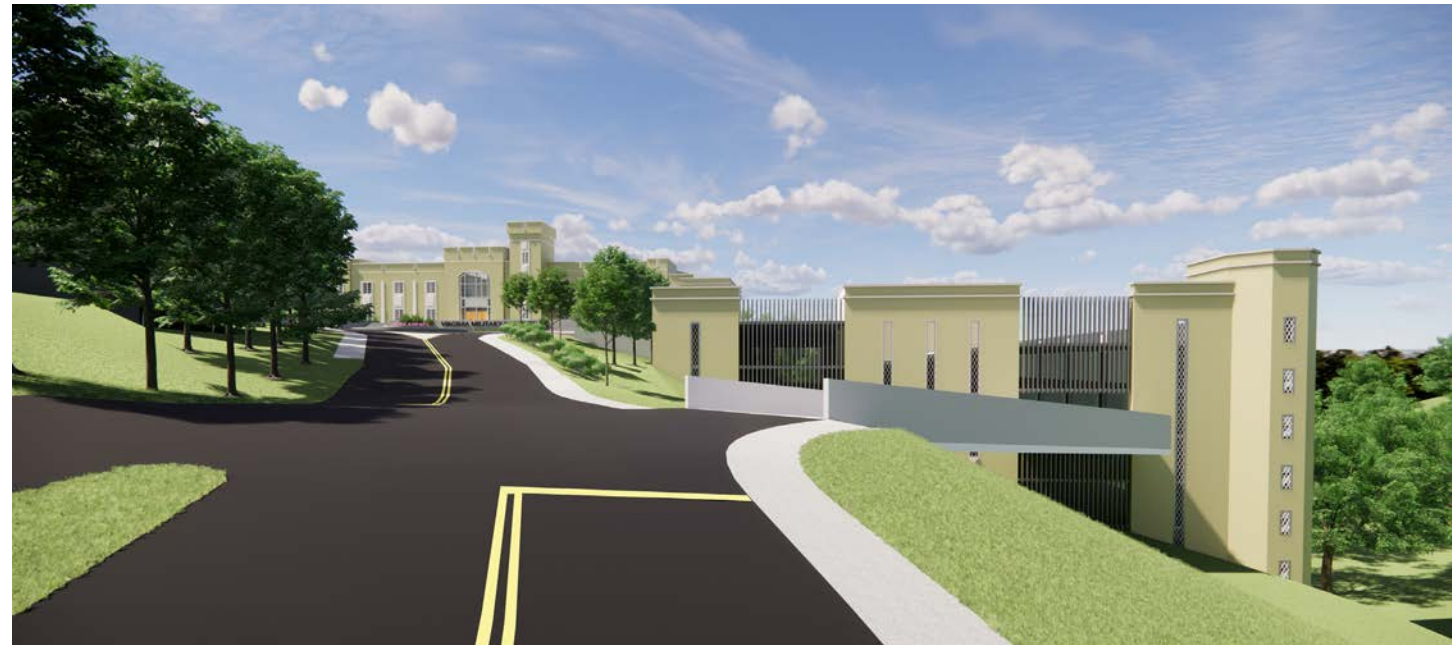
▲ The upper-most parking level entry will be at the level of the roundabout and continue down from that point.
