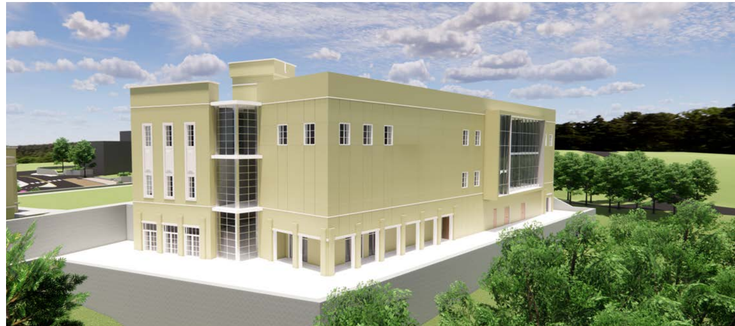
▲ Sections of floor to ceiling glass allow views to nature.
