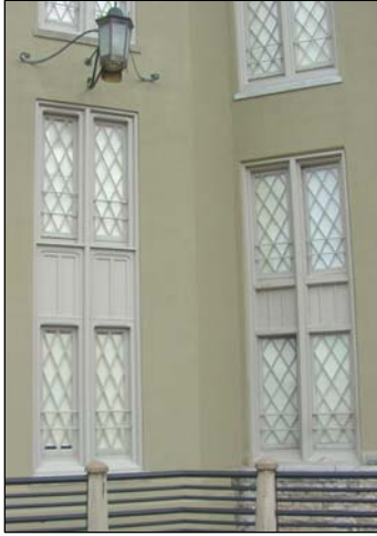
Historic windows have been maintained and preserved at the Barracks.
