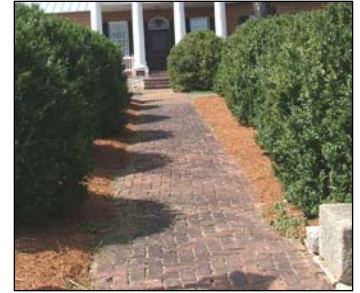
The pedestrian walk leading to Stono is constructed of dry-laid brick in a herringbone pattern.
