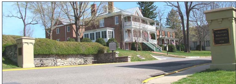
View of South Institute Hill shows landscape structures in good condition, including the historic Limit Posts.
