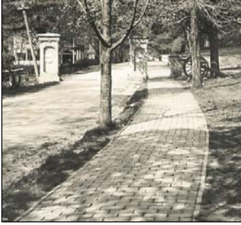
1925 image shows Lexington brick sidewalks which have since been replaced with concrete sidewalks.
