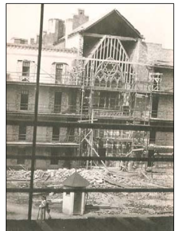
1916 image of demolition of Jackson Memorial Hall and Barracks project.
