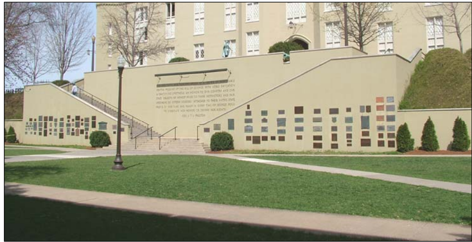
The Memorial Garden (1927) is one of the most prominent open spaces on the Post; the monumental staircase on the north edge includes memorials and leads to the south side of the Old Barracks.
