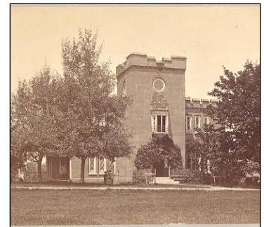
Rebuilt Officers’ Quarters.
