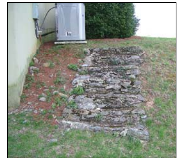
Stacked and mortared stone at 410 VMI Parade is in poor condition.
