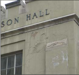
The use of stucco is evident throughout the Post, as seen here at Richardson Hall.
