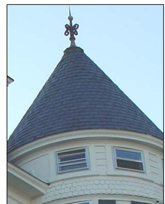
320 Institute Hill has a slate roof.
