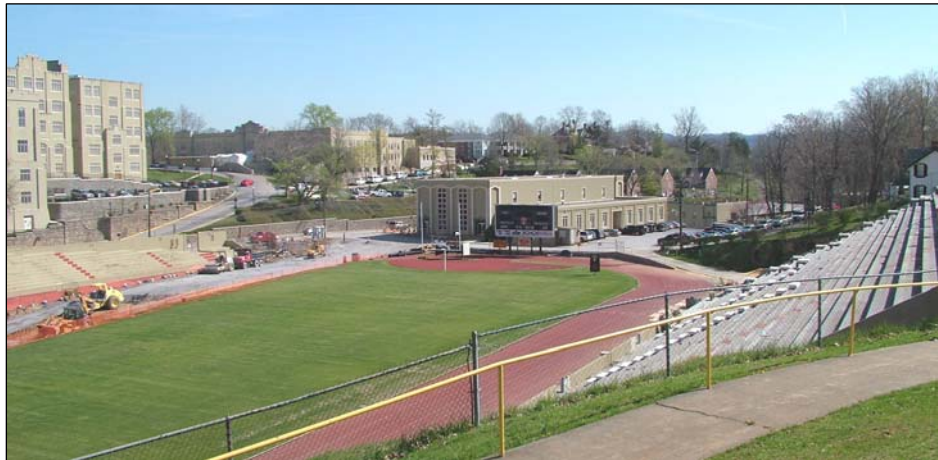
View from South Post looking towards Central Post.
