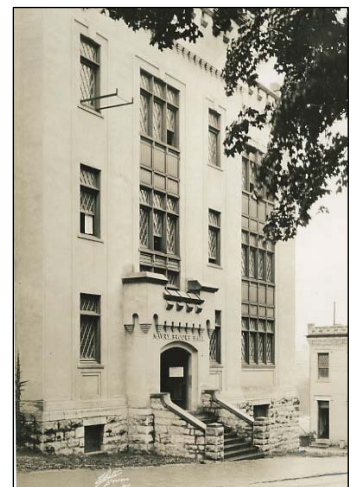
Maury-Brooke Hall, shown here in 1925, was constructed in 1909.
