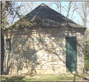
A wood shingle roof is used on a Stono outbuilding.
