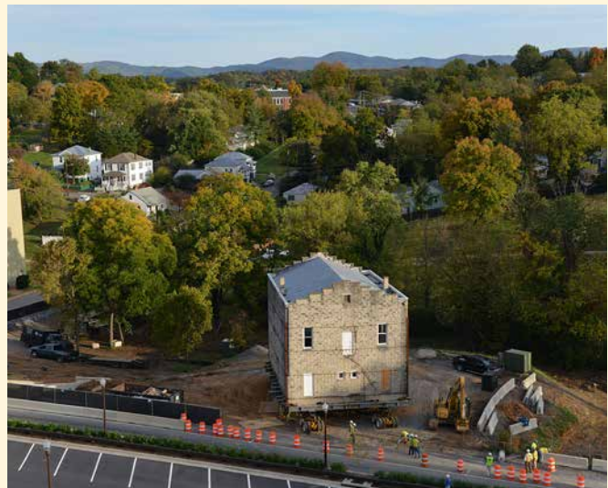
In 2014, the Knights of Pythias building moves to its new location along Main Street to make room for the Corps Physical Training Facility.—VMI File Photo by Kelly Nye.
