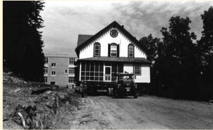
The Pendleton-Coles House, now home to the Office of Admissions, is moved to make way for the construction of Maury-Brooke Hall.—Photo courtesy of VMI Archives.
