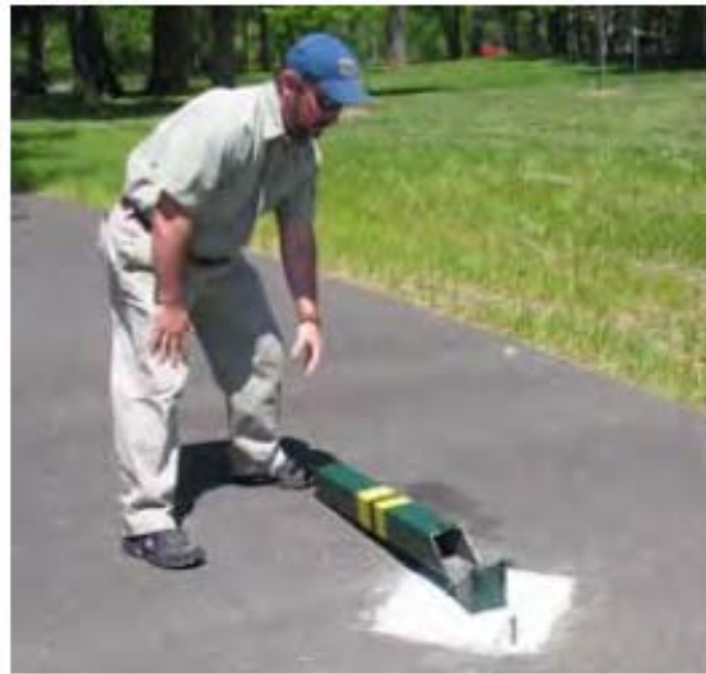
Vehicles can drive over collapsible bollards without completely removing the bollard from the ground. Courtesy of Roanoke Valley Greenways.
