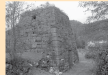
The remains of the Glenwood Furnace can still be seen beside Virginia 750 in Amold's Valley near Natural Bridge. It is typical of the foundries which once dotted the region.
